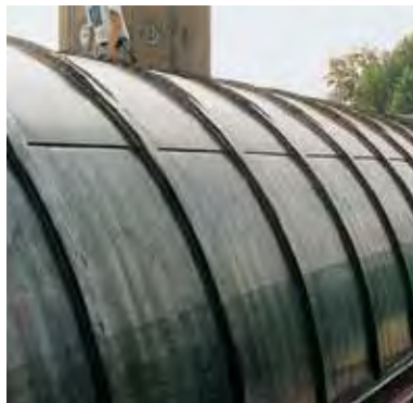
The sides of the sheet metal which are bent up are seamed together using a cover plate.
