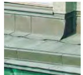
A wide facade moulding fitted with a gutter to allow water to run off. Mouldings of this kind are made in the same way as roof coverings.
