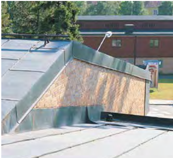
A cover flashing lying parallel to the pitched roof area. The cover flashing can move freely in relation to the connecting wall because it has been attached using hook bolts. The cover moulding protects the connection.
