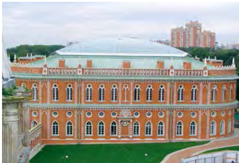
Large areas of Long Strip roofing, created with Nordic Green pre-patinated copper, are used throughout the Tsaritsyno Palace in Moscow.
