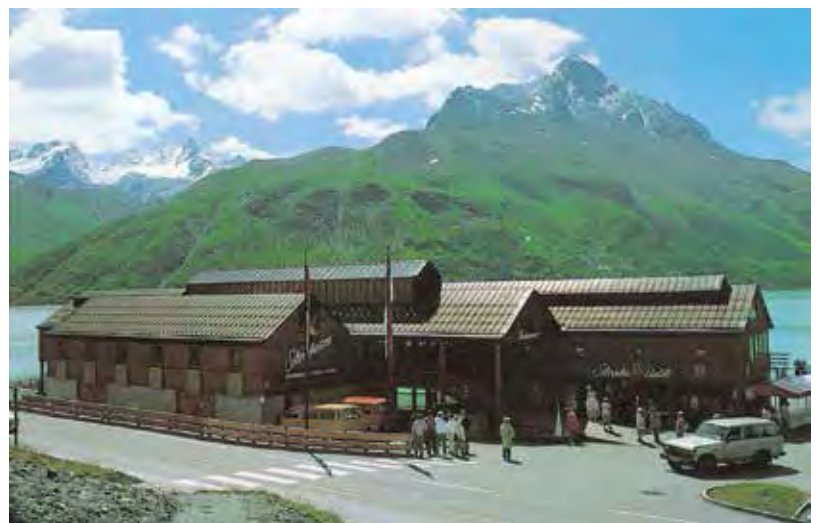
Snow slide guard over an entrance.
