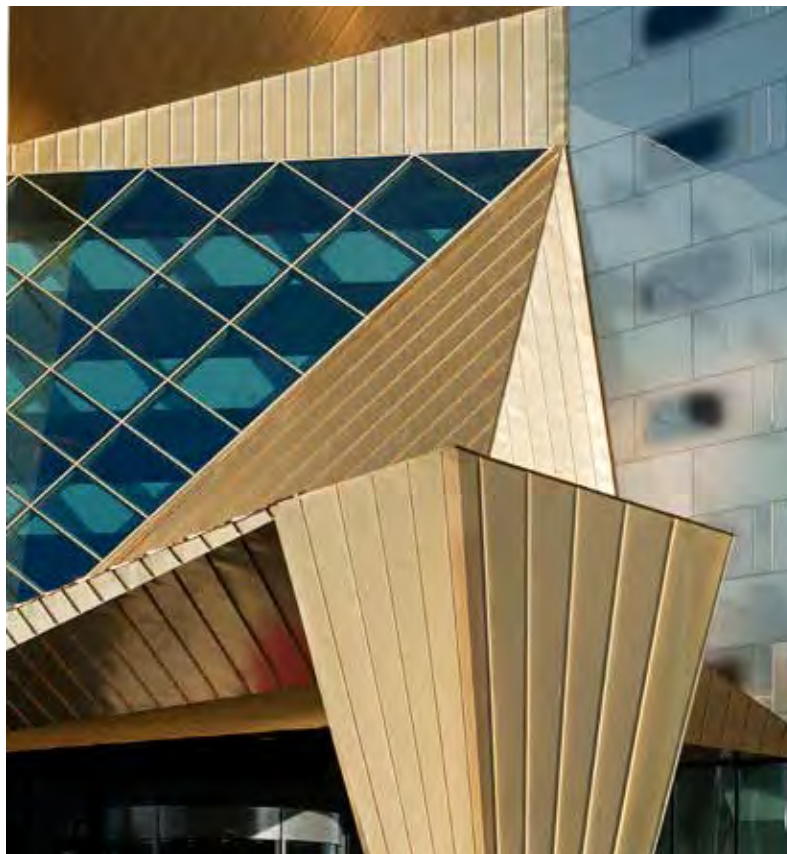
Examples of standing seam.
