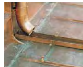
Is the downpipe union piece attached to the wall?
