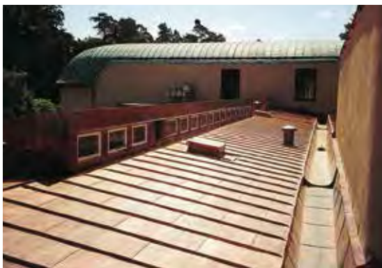
A beautiful roof is worth maintaining.
