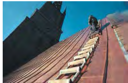
Steeply sloping roof.
