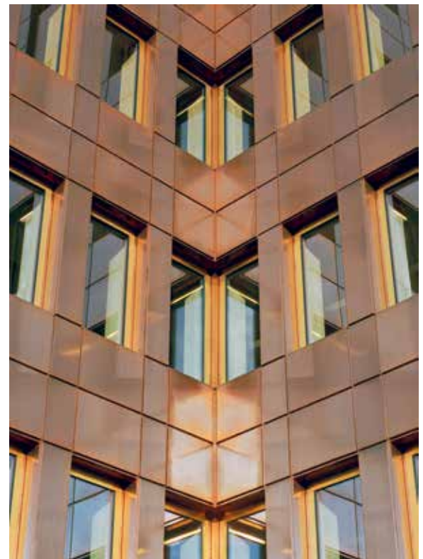
Copper cassette facade on office building in Skellefteå, Sweden.
