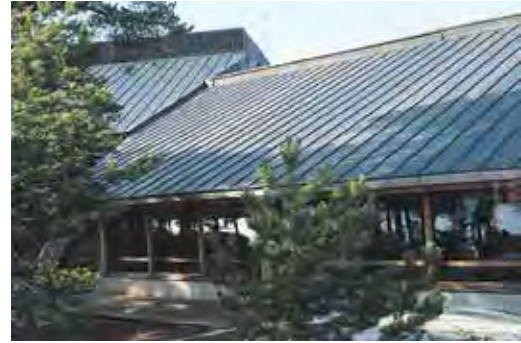
Roof with no obstructions.
