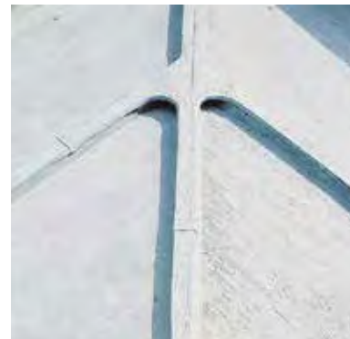
Examples of batten roll.
