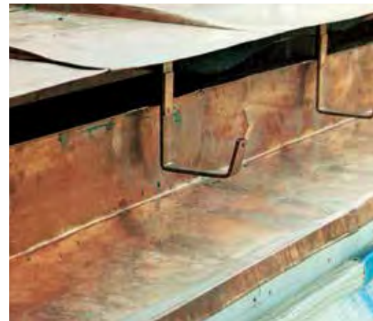
Example of protective flushings (gutters not yet installed).
