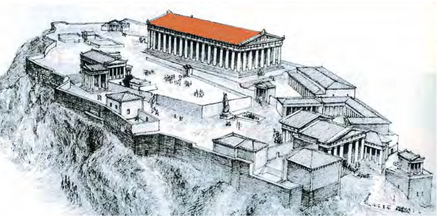
Scientists have reason to believe that the roof of Parthenon Temple Acropolis, Greek (448–432 BC) was made of small copper sheets.
