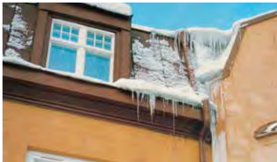
Stresses caused by ice on the eaves, box gutter and downpipe.
