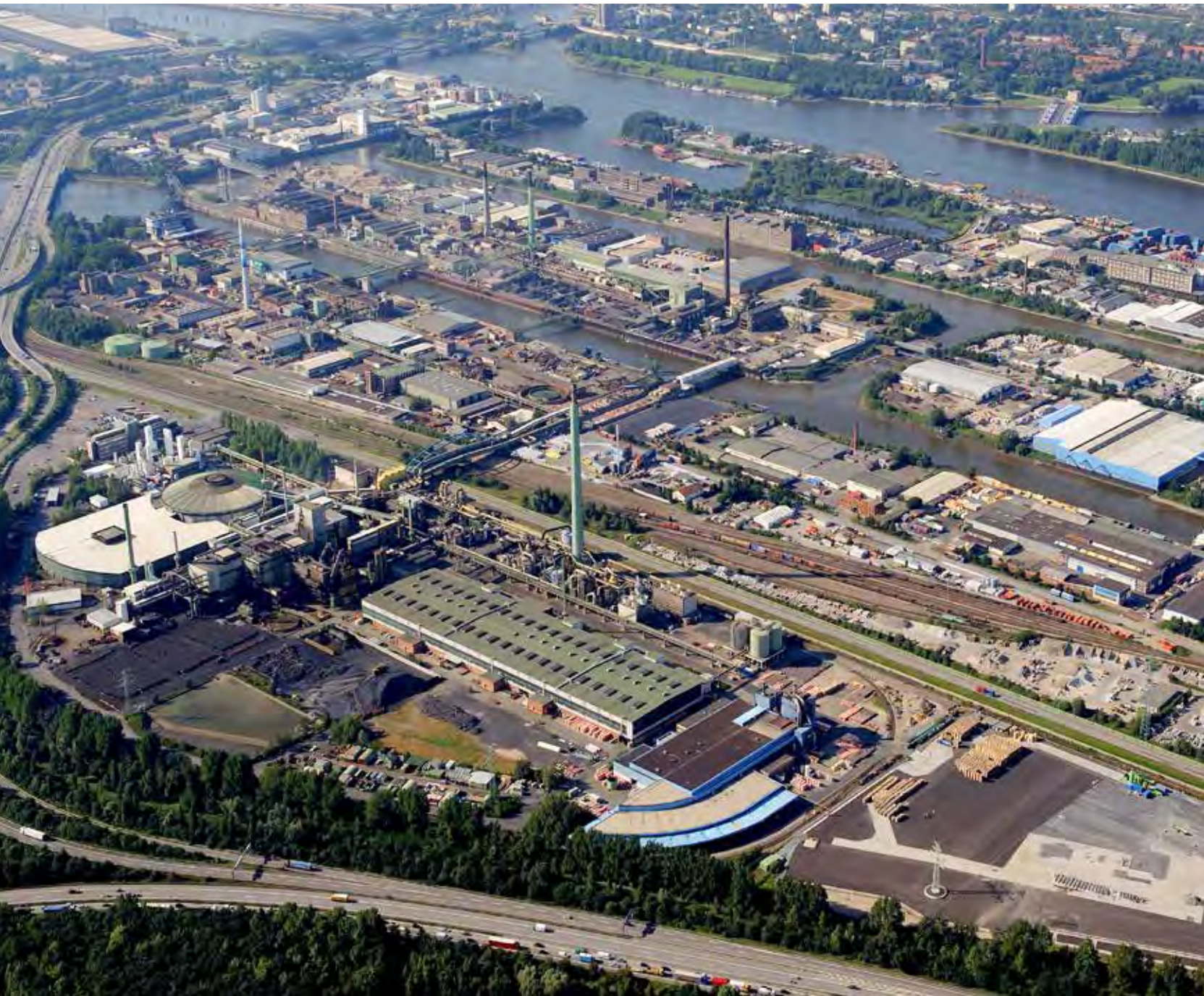
Aerial photo of the Aurubis headquarter in Hamburg, Germany.
