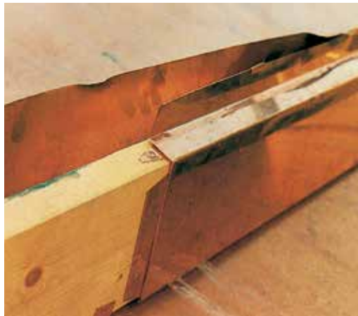
A timber frame is used for gutters for copper coverings.
