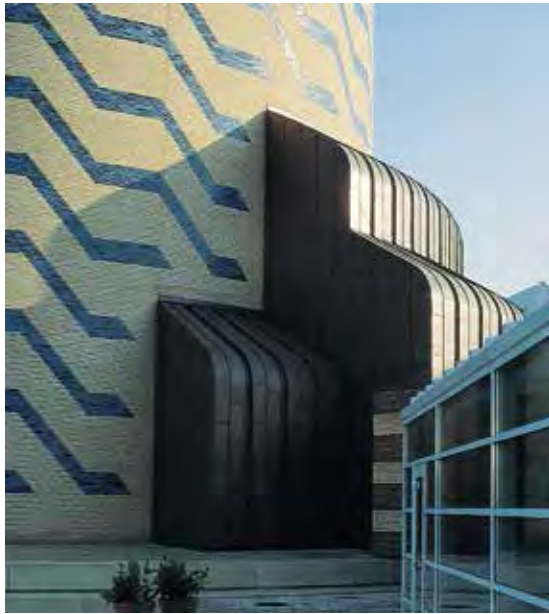
Flat sheeting is a good material for curved surfaces. Planetarium in Copenhagen, Denmark.
