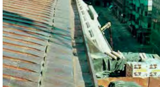
Valleys – including gulleys – are some of the most important details of a roof and must be checked and maintained with precision. They should be cleared of snow in the winter, and this must be done carefully so as to avoid damaging the roof covering – use a wooden shovel.
